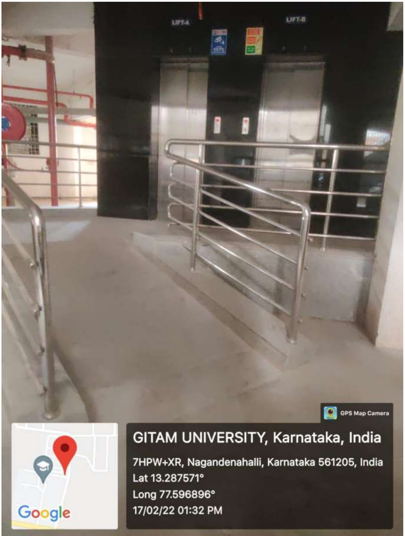
Ramp Facility in the Building
