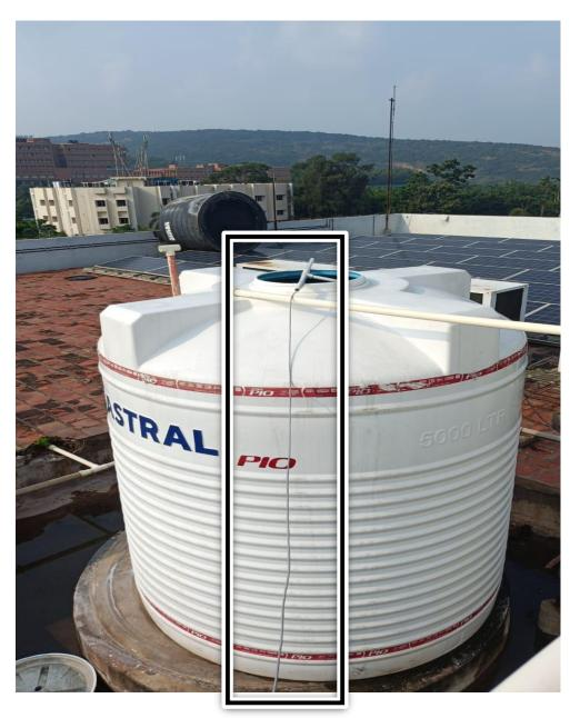
All the water tanks are equipped with IOT tool to sensor the water level filled and auto terminate the inflow, which is monitored and controlled by using a App
